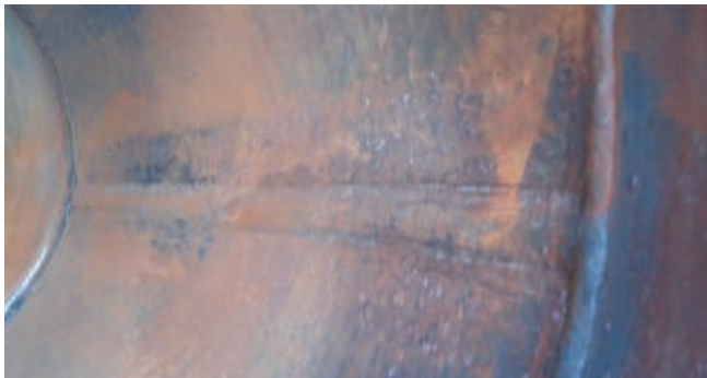
The internal surface of this meter tube shows signs that it was not protected by a non-toxic vapor phase corrosion inhibitor (Fig. 4).
