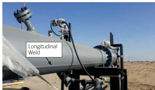
Pipes used for the downstream meter tube had longitudinal seam welds (Fig. 1).
