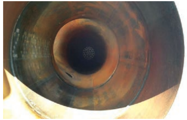
This same meter tube shown in Fig. 4 also has internal circumferential girth welds not ground flush with the pipe wall (Fig. 5).
