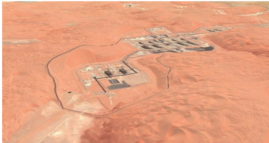
The Shah gas development geographically separates low-risk areas of the plant from higher-risk areas containing high-pressure, toxic fluids (Fig. 5). Photograph from Al Hosn Gas.
