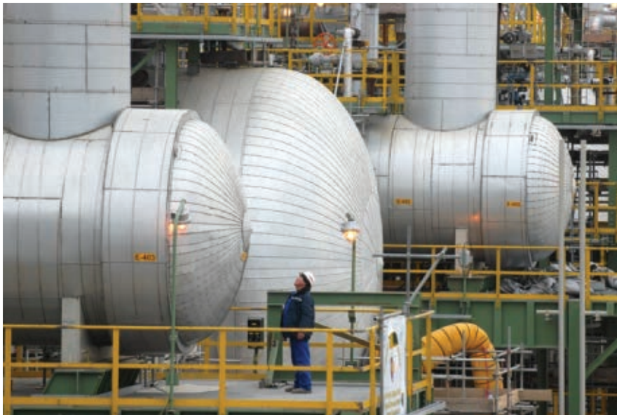
The Tengiz SRU features a 328-tonne, first-stage sulfur condenser (Fig. 3). Photograph from Tengizchevroil.
