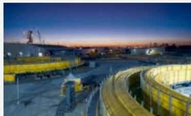
Aker Solutions’ umbilical facility in Mobile, Alabama, with its high-capacity horizontal cable, is specially designed to meet the challenges of demanding deepwater applications.
