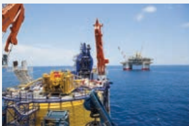
McDermott's North Ocean 102 installed umbilicals totaling 65 miles.
